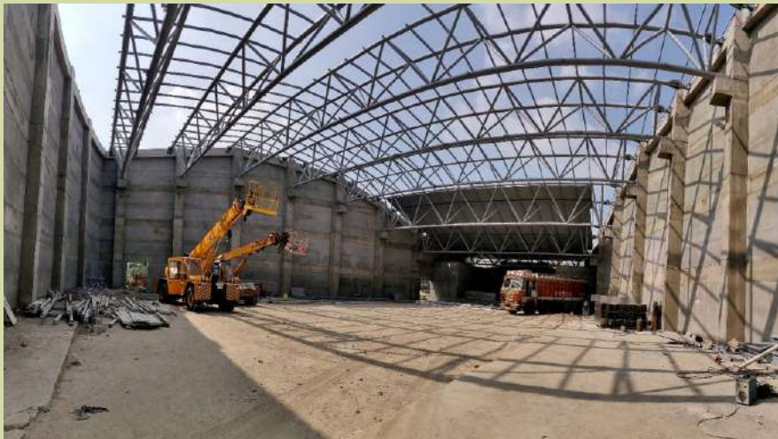
'V' truss span increases from 20m to 43m to facilitate a column-free space for a multi-purpose hall.
