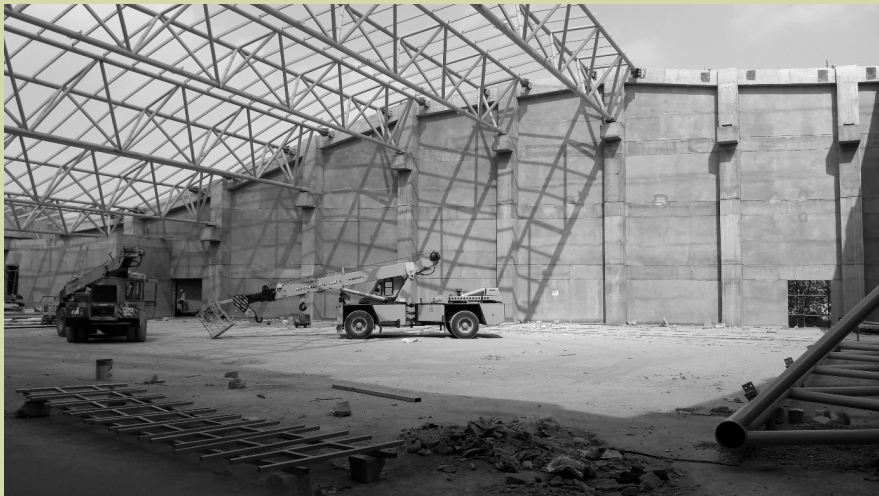
'V' truss span increases from 20m to 43m to facilitate a column-free space for a multi-purpose hall.
