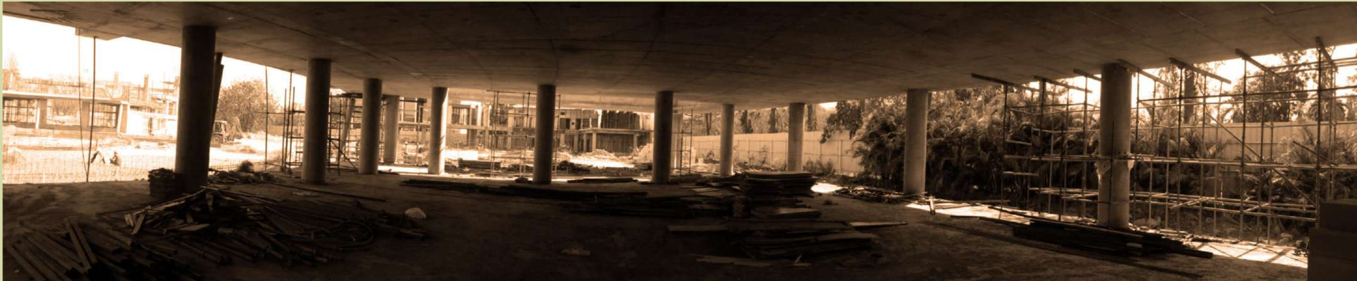
23m column free Post-tensioned (PT) span in expose concrete.
