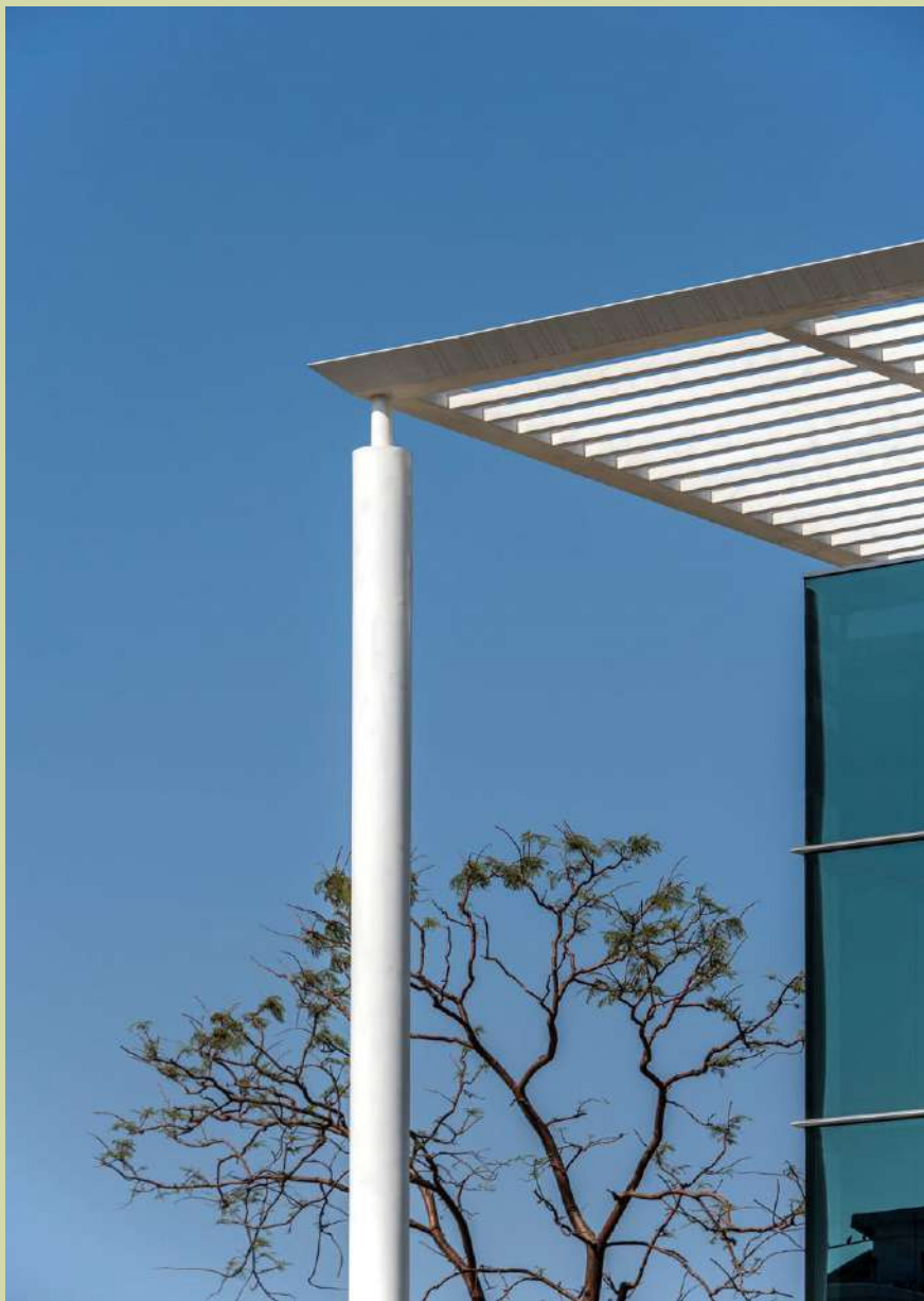
A pin joint coloum holding 9.5 m x 9.5m canopy.
